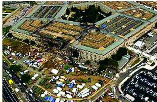
Above: Aerial view of the Pentagon showing the Phoenix, the collapsed section of the building. Photo taken on September 14, 2001 by the Department of Defense.
